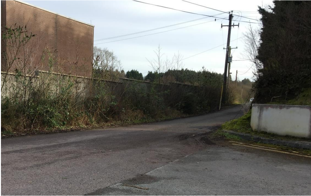
Figure 12: Inadequate sightlines at Berkley road and Templegrove junction
